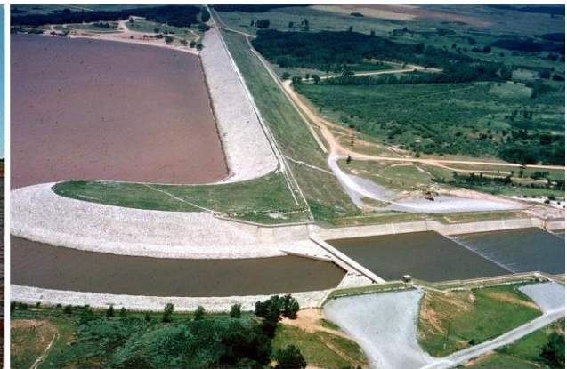
Aerial view of new dam & spillways
