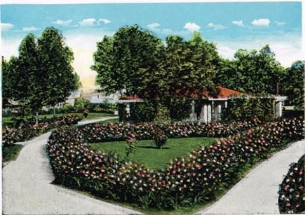
Pagoda in Court House Square.
