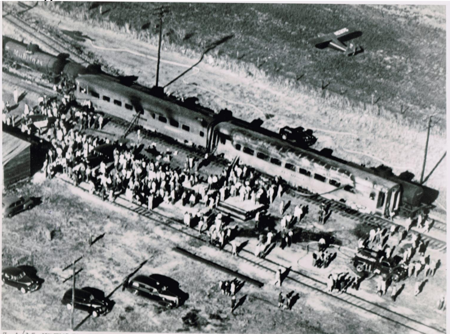
3-4/15-KREMLIN, OKLA: Fire hoses snake their way from fire truck (lower rt) to 2 cars of Rock Island Texas Rocket after streamliner was hit by a truck & ear cars left rails & skidded along parked oil cars on siding at Kremlin, a. Note paint scorched from cars, fire ladder in window at left & ambulance foreground. At least 2 were killed, 20 injured in wreck. (ACME TELEPHOTO)
