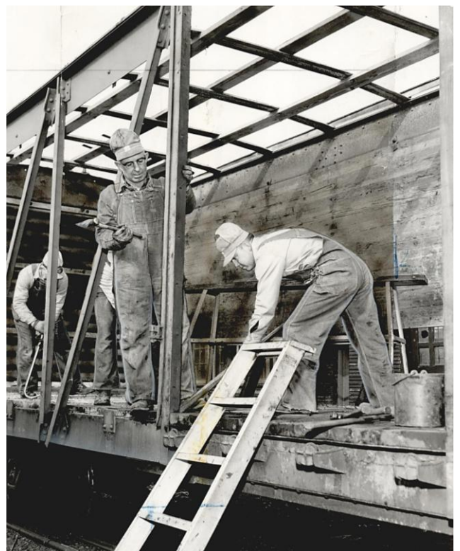
Boxcar undergoing repairs on a riptrack (repair in place track) at the Frisco railyards in Enid OK in 1958 . Riptracks are sidings in railyards where repairs can be done "in place" without transferring damaged cars to repair sheds. The boxcar shown is undergoing relatively major repairs.
