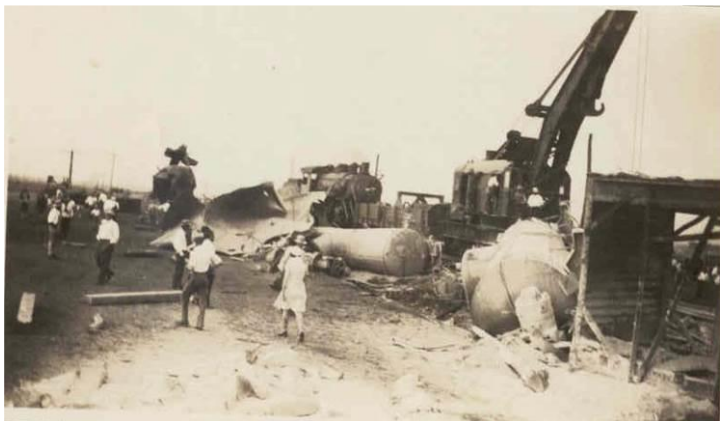
Above, L & R: Railroad crane removing debris, including tank cars, from the wreck site. Note the steam engine of the salvage train in the l photo, probably looking S.
